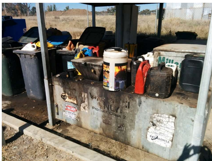
Figure 7 roofed and bunded waste oil disposal point
