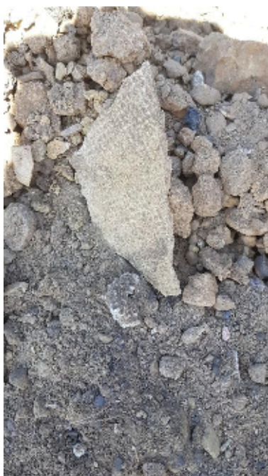
Waste containing asbestos Photos by Mike Haywood
